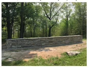
So what we ended up with is Susan's Wall! It is 30 feet long, just a little under two feet wide and three feet in height, built on a slight arc. It is made of Perth sandstone, quarried in the 1860's at Hughes Quarry just off Elmgrove Road, to build the stables at the old bank building that stands at the corner of
